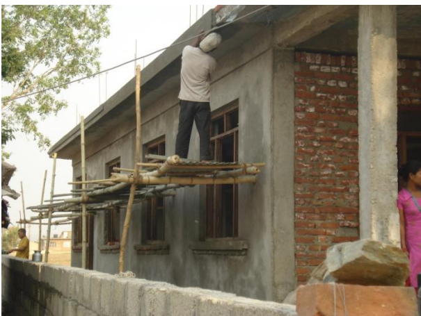
The building work continues at a pace.
